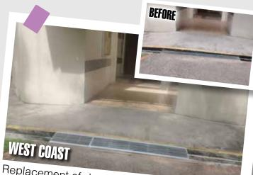
Replacement of damaged grating near to Lift C of Blk 712 Clementi West St 2
